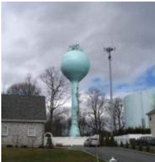
Elevated and Ground Storage Tanks at Schoolhouse Place
