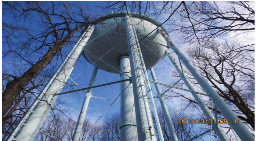
Mill River Road Road Elevated Water Storage Tank
