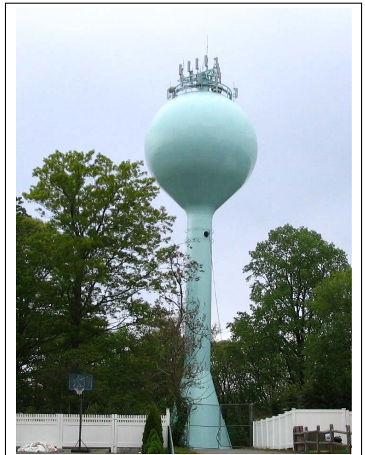
Schoolhouse Place tank after rehabilitation and repainting project.
